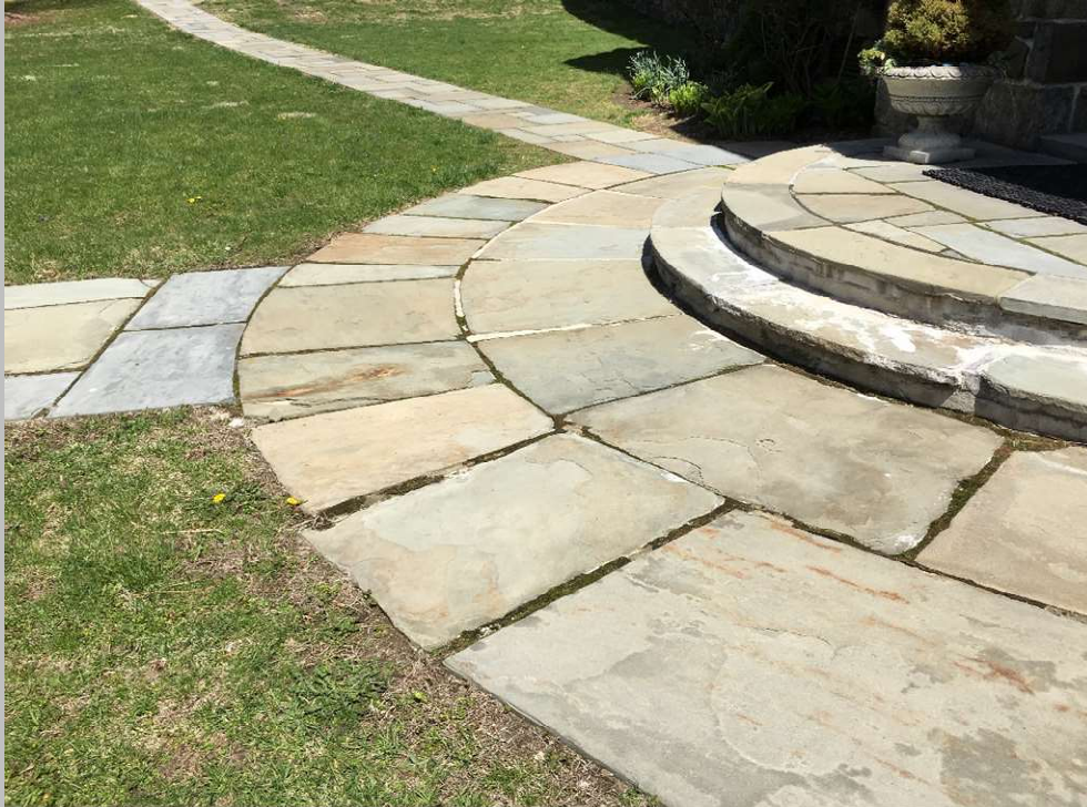
Main Entrance Steps/Walkways
