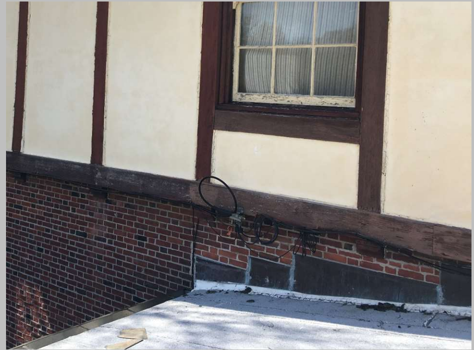
Wood Facade Repair
