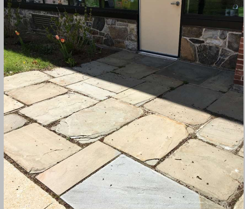
Main Entrance Steps/Walkways
