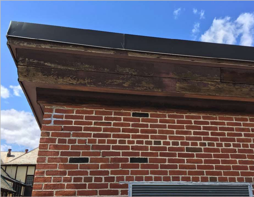
Wood Fascia Replacement
